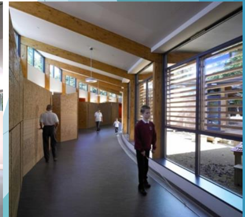
Cork tiles at corridors
